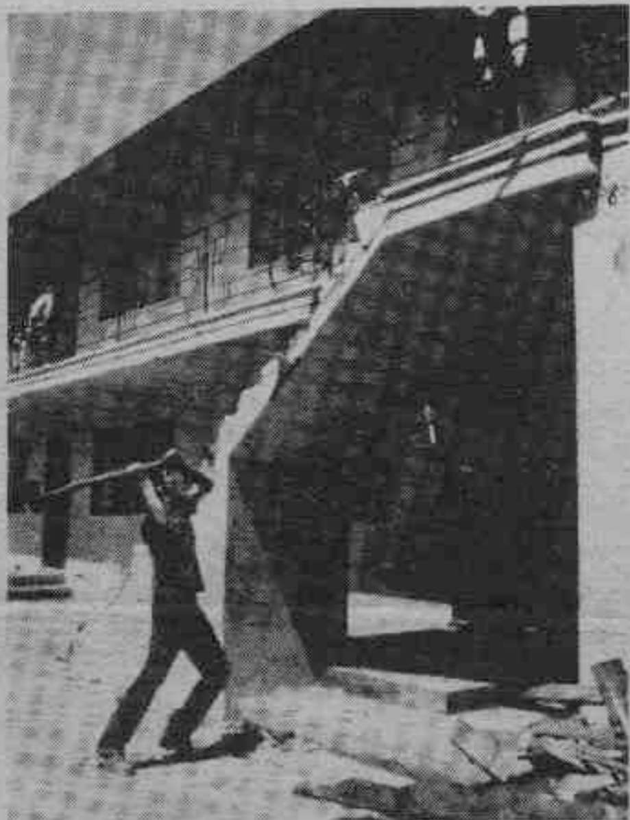
TENANTS DEMOLISH STAIRS AT CCSM'S 20TH ST. BUILDING
