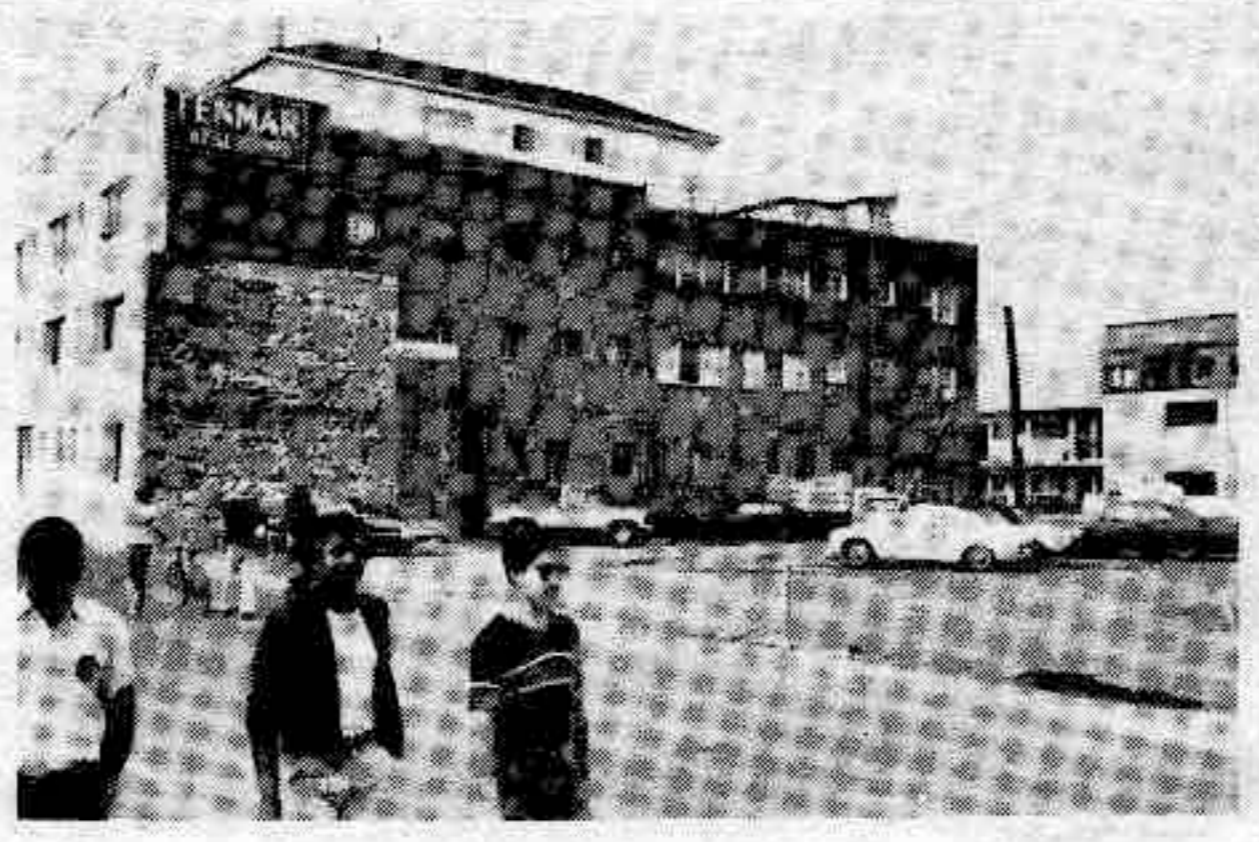
Breeze Ave. lot now site of SeaBreeze Project.
