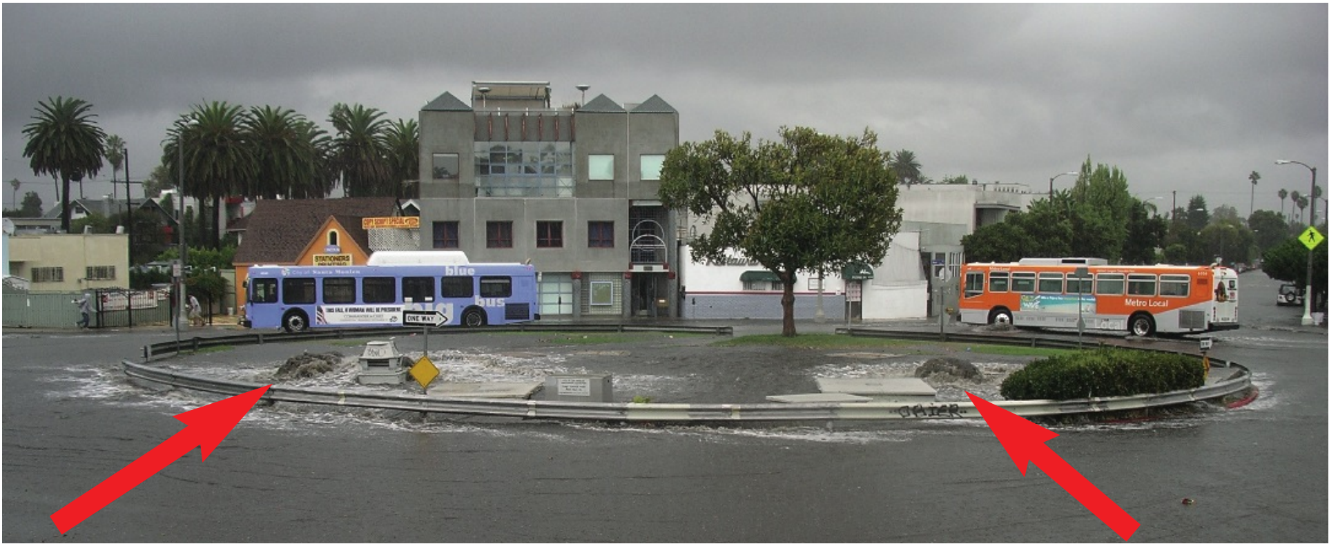
An October 17 cloud burst brought back knee-deep canals in the former lagoon (now Circle) and surrounding streets. The storm drains (see red arrows) overflowed and created dirty-brown fountains in the Circle. Surely an improvement over the “landscaping” the city of L.A. thinks we need.
